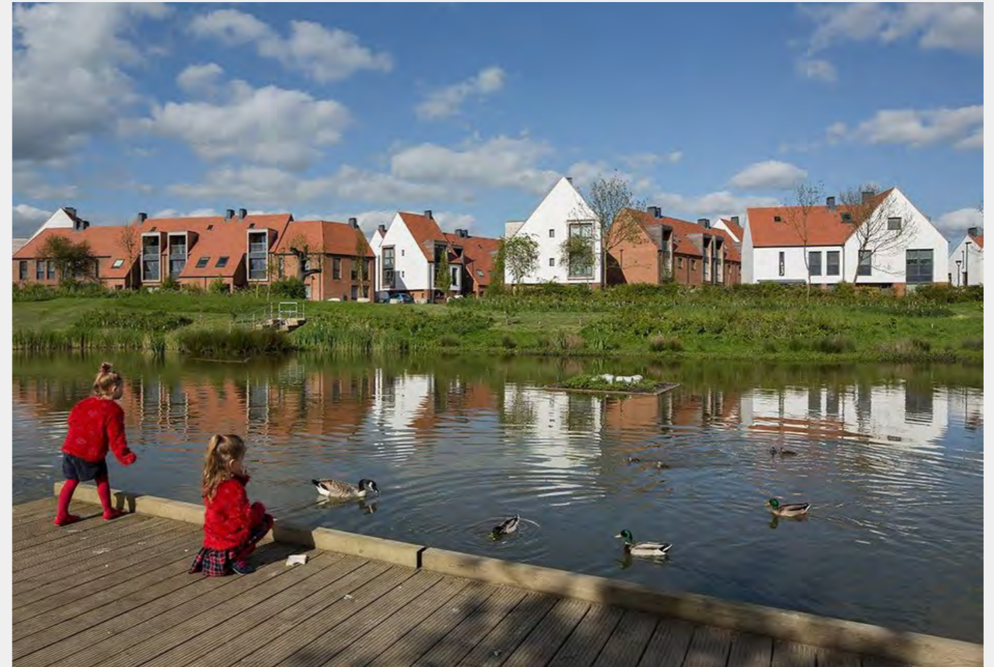
Derwenthorpe fase 1, Osbaldwick (Eng), Studio Partington
